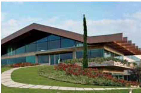
Dasty Italia SpA head office and production facility, Bergamo, Italy.
